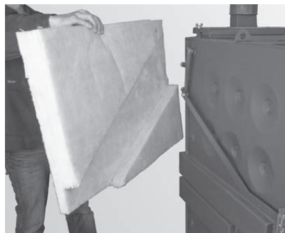
Fig. 43 Monter les isolations (LogWIN Klassik pellet ready)
